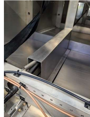
Pushrod cover installed
