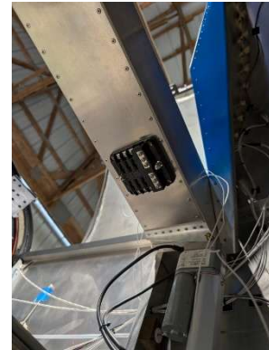
Aux fuse box installed
