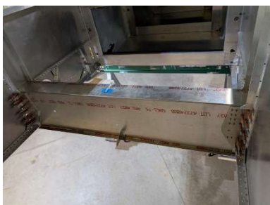
Forward tunnel zee clecoed to side panels
