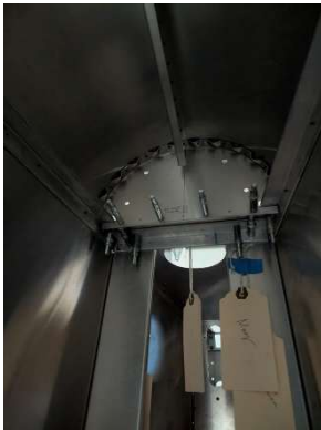
Inside view of former #5
