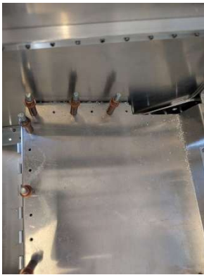
Seat pan temporarily installed and holes transferred to support angles
