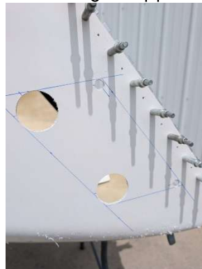
Holes drilled for corners
