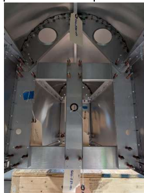
Aft fuselage station #4 updrilled
