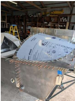
RH side longeron holes updrilled
