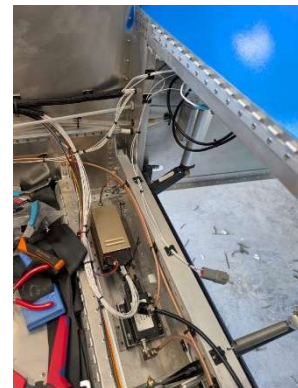
Smoke system harness wired
