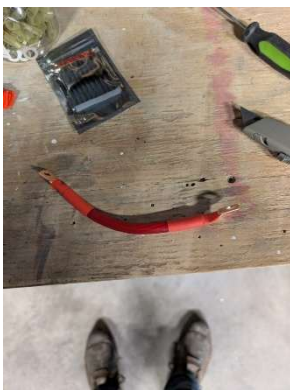
Cable from battery to master relay
