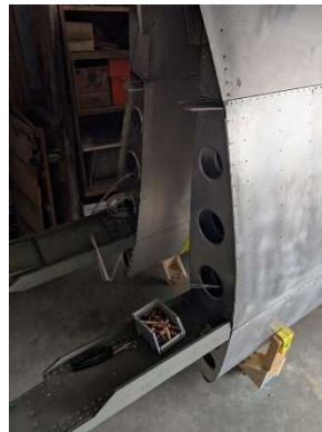
Wing doublers removed
