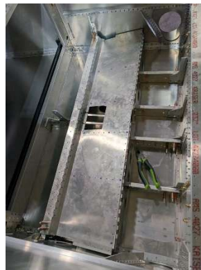
Rear seat pan reinstalled. Temp blue rivets used to pin alignment
