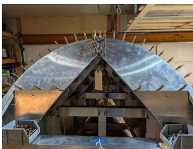
Former #1 updrilled including splice plate
