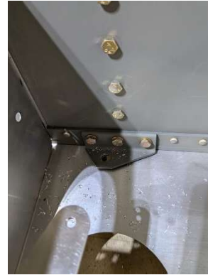
Tie down bolt hole drilled
