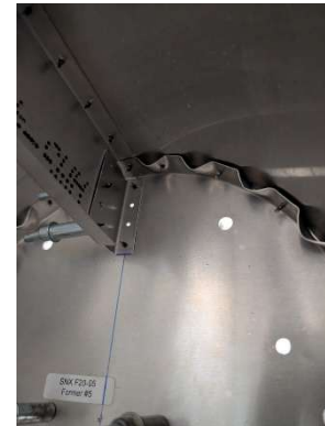
Aft clip located and pilot drilled to skin splice channel and former #5
