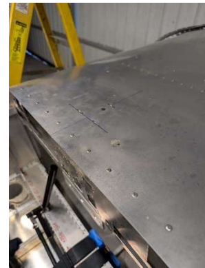
Nutplates and grommet installed
