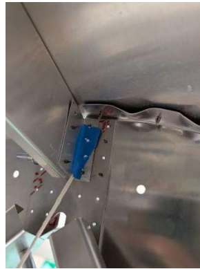
Forward skin splice channel clip located and pilot drilled
