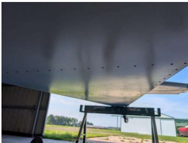
Aft fuselage floor riveted
