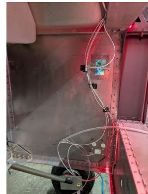
Fuselage side harness securement laid out
