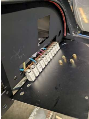
Connecting wires to circuit breakers
