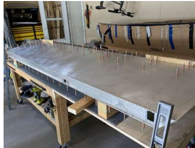
RH upper aft wing skin riveting in progress
