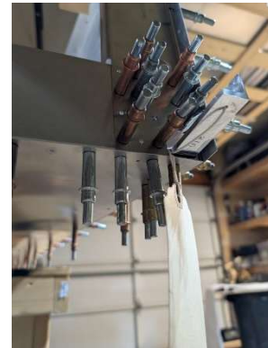
Holes drilled through spacers, lower splice plates, lower crossie, and aft fuselage floor
