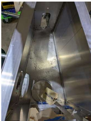
Aft shear Web assembly aligned
