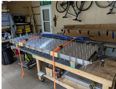
Setting lower forward skin with ratchet straps
