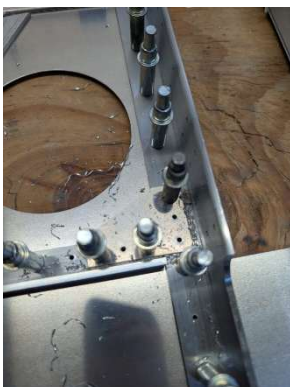
F14-10 gusset located and pilot drilled
