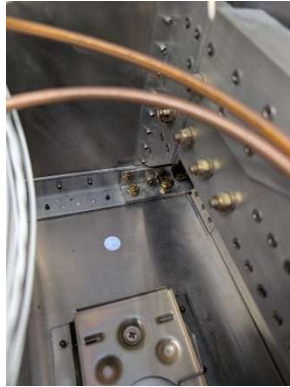
Splice plate bolts installed
