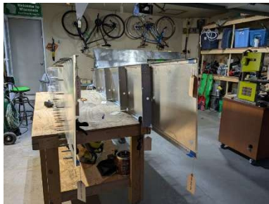
Vertical channels installed
