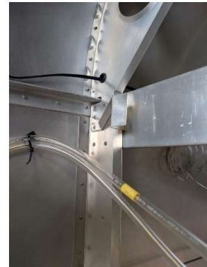
Support bracket riveted to #2 vertical channel
