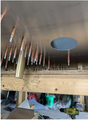
Pitot mount doubler holes drilled
