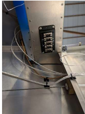
SkyView splitter installed
