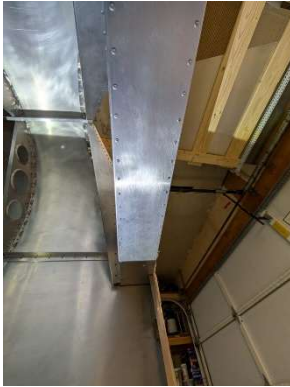
Crosstie closeout riveted into place
