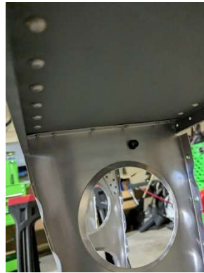
#5 forward rib installed
