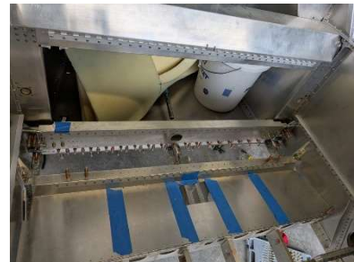
Rear spar carry through progress
