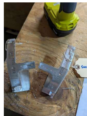
Holes drilled in horizontal sides of splice plates
