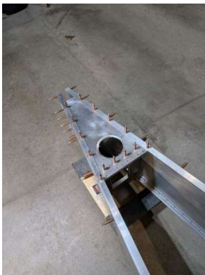
Aft shear web assembly fit
