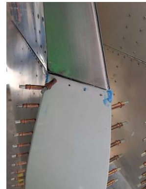
SuperFil being applied to damaged fiberglass
