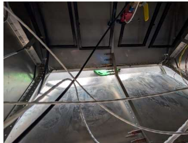
Brake lines connected to center tee fitting
