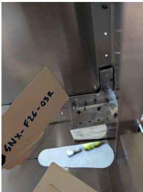
F22-07 spacers inserted and pilot drilled
