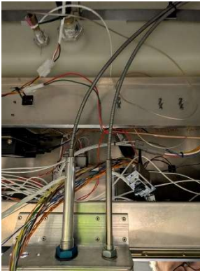
Mixture cable installed
