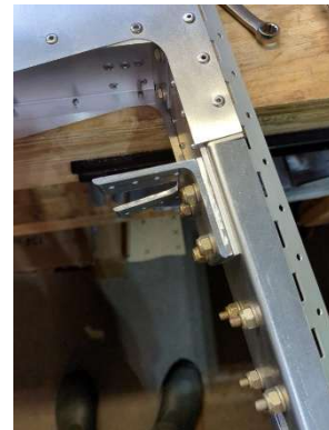
Temporary spacer installed
