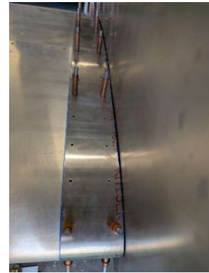
RH wing root doubler clecoed into place
