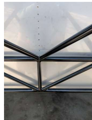
Bulkhead fitting marked per plans
