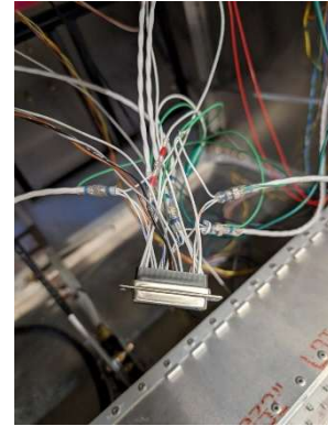
Finished populating intercom harness
