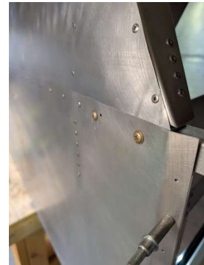
Bolts in upper splice plate installed
