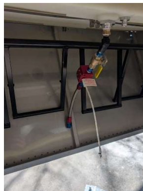
Fuel system plumbing in progress
