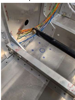
Marking com antenna mounting holes
