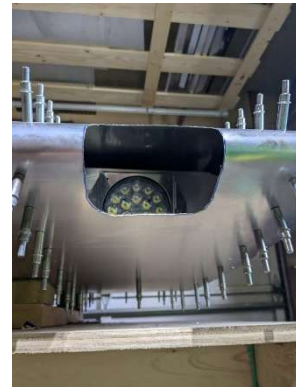
Opening rough cut
