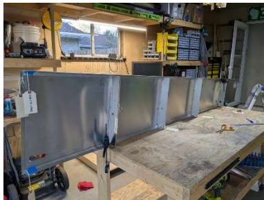
Vertical channels 2-5 installed on RH panel
