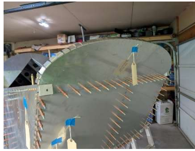
Upper firewall updrilled
