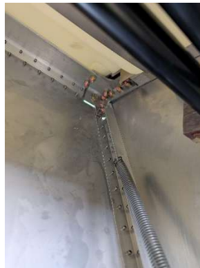
Upper motor mount bolts installed and torque check applied
