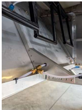
Forward floor stiffener riveted
