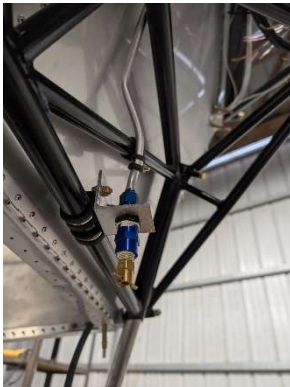
Drain line complete (minus leak testing)
