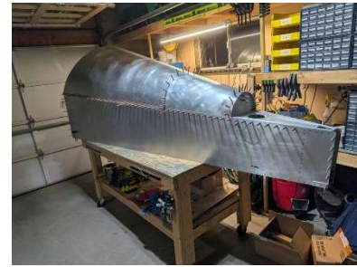
Formers #5 and #4L/R clecoed into place
