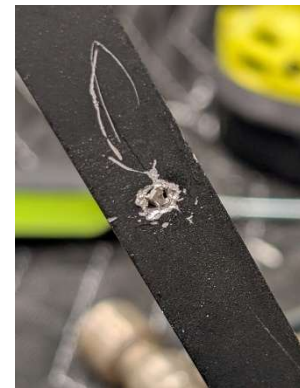
Broken tap in aft canopy frame
