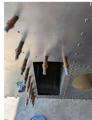
Spar tunnel top angle brace holes transferred and updrilled
