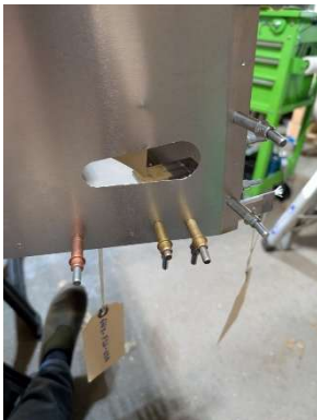
RH bolt holes through lower splice plate
