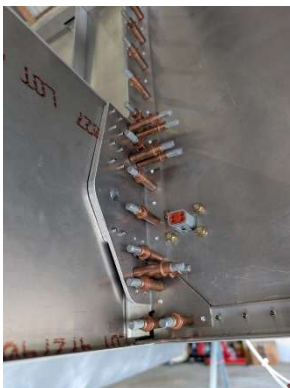
LH bulkhead connector installed
