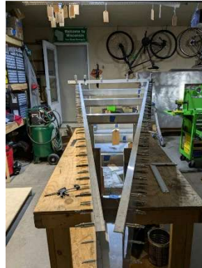
Upper and lower cross ties fit, pilot drilled, and clecoed
