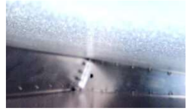
Interior of rudder
