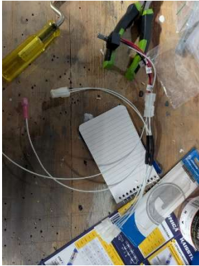
Panel lights harness fabricated
