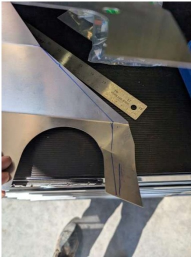
Marking trim lines for cylinder baffles
