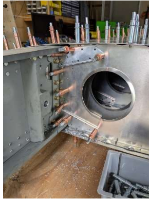
Aft root rib attach angle updrilled
