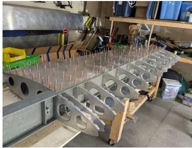
LH wing skin installation in progress
