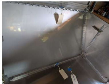
Lower firewall located and pilot drilled
