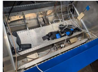
Antenna cables routed and secured
