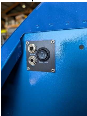
Seat heat switches installed
