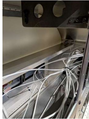
Sub-panel test fit
