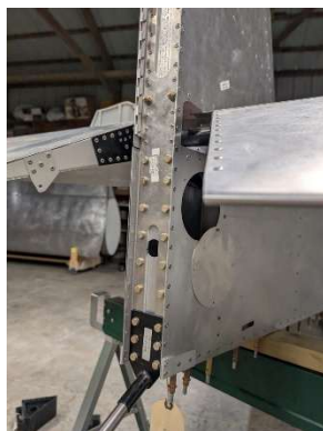
Rear stabilizer bolts installed
