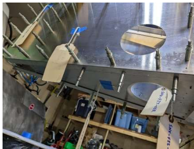
Aft shear web assembly pilot drilled and clecoed
