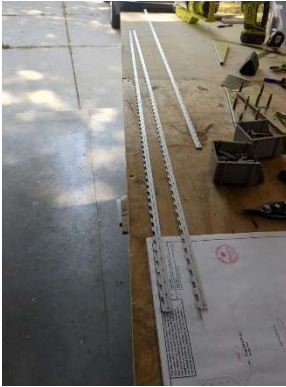
-06L/R hinge halves cut and pilot drilled
