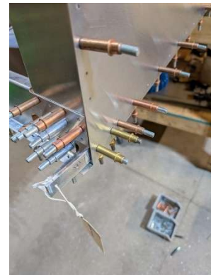
AN525 bolt holes drilled in lower splice plates
