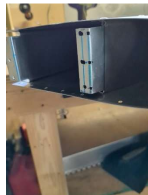
Hole issues fixed with doubler plate
