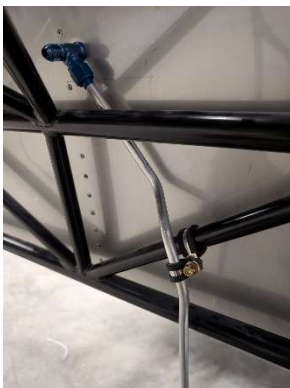
Bending and test fitting drain line
