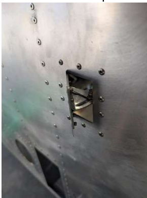
Vent assemblies complete
