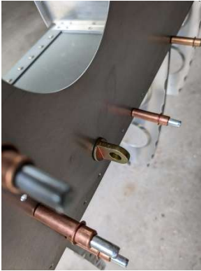
LH tie down bolt torqued
