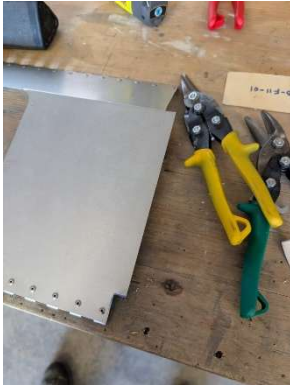
Trimming lower seat pan
