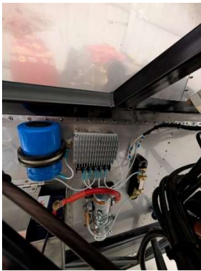
Voltage regulator wiring mostly complete
