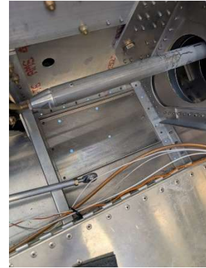
Stiffener installed and mounting holes drilled
