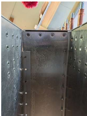
Side clips installed with flush rivets
