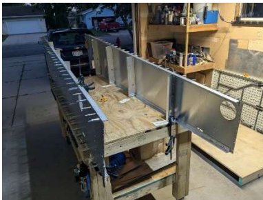
Vertical channels installed
