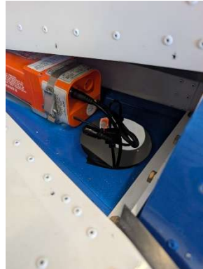
ELT wiring secured in tail cone
