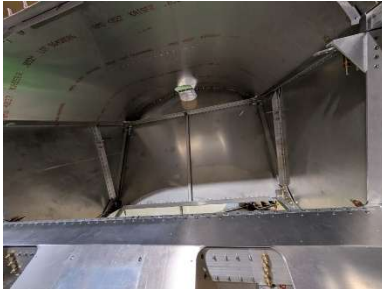
Glareshield riveted to longerons
