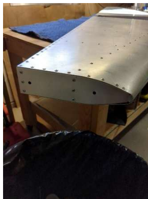
Removal of tip rib to attach mount doubler
