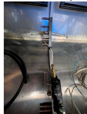
Master cylinder installed and main brake line plumbed
