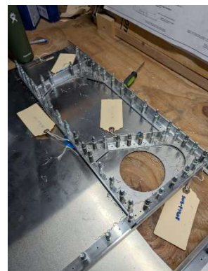
Misc. Gussets located and pilot drilled
