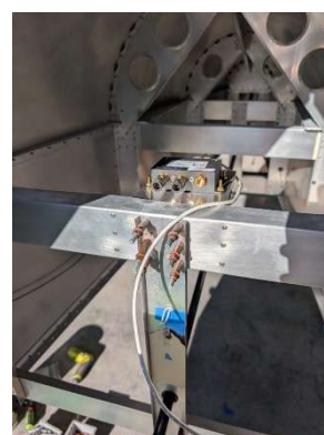
SV-ADAHRS-200 until installed and test cable ran
