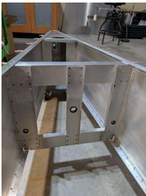
#4 cross ties riveted
