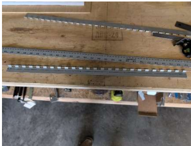
Canopy hinge cut and pilot drilled
