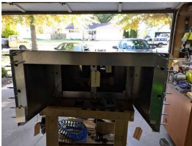
#1 lower cross tie located, pilot drilled, and clecoed
