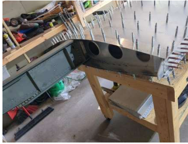
Aft root rib fitted
