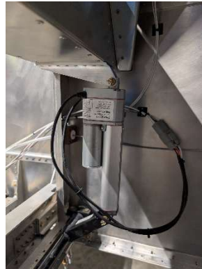
Flap motor hardware installed
