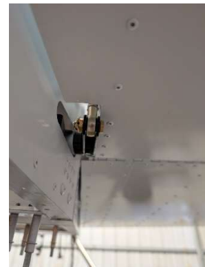
RH flap hardware installed
