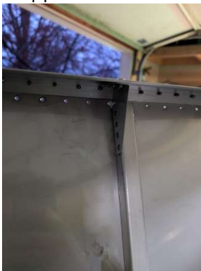
Firewall Stiffener and upper angle riveted
