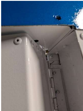
Rudder cotter pin holes drilled and pins installed
