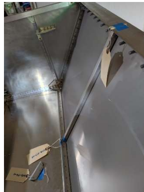
Firewall stiffener pilot drilled
