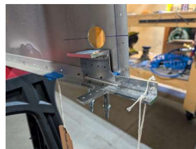
LH lower splice plate pilot drilled
