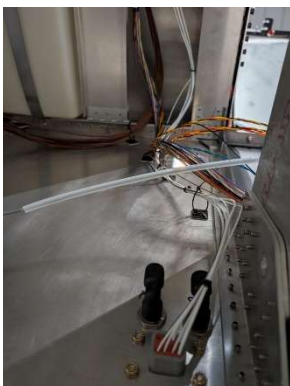
Engine sensor harness installed
