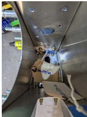
Drilling AN3 holes into aft support angle
