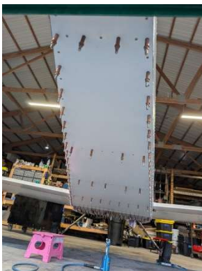
Aft fuselage floor riveting began
