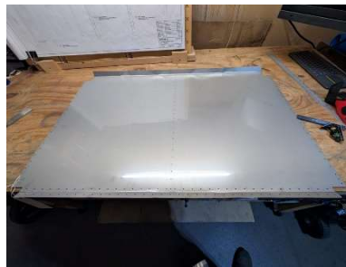
Bending up ends of -01 lower firewall
