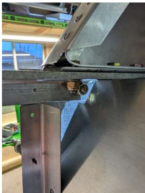
RH splice plate bolts
