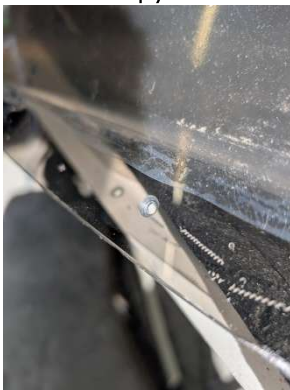
Deburring and countersinking canopy holes
