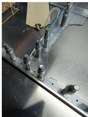
F14-10 gusset located and pilot drilled
