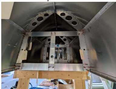
Aft fuselage station #2 updrilled
