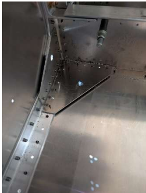
LH gusset and spacer located and pilot drilled
