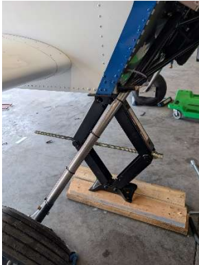
RH gear bolts replaced with NAS bolts
