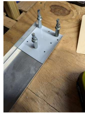
Using template to drill holes
