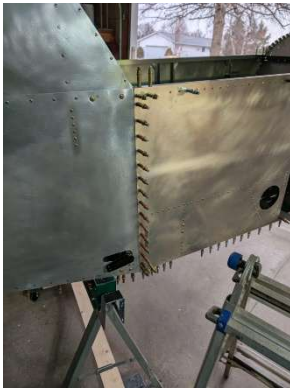
RH side panels updrilled
