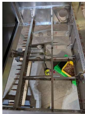
Floor removed and components updrilled
