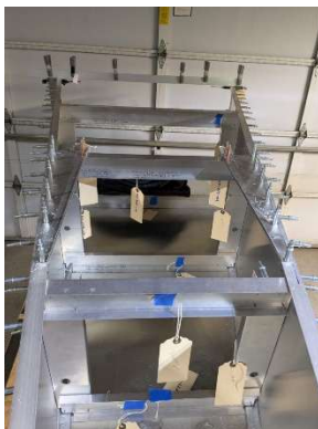
Both aft angles fit and pilot drilled
