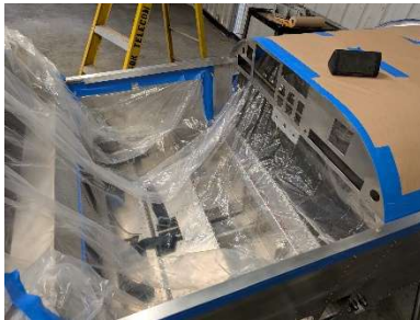
Drop cloth fit in cabin area
