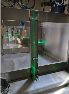
Forward push rod support located and pilot drilled
