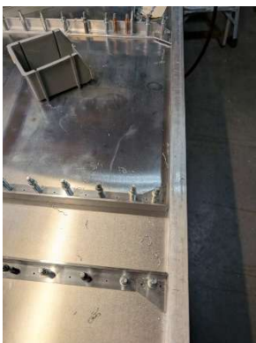
F14-10 gussets located and pilot drilled
