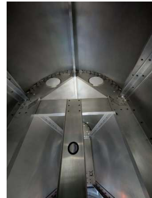
#4 formers riveted to tail cone box and skin splice channel
