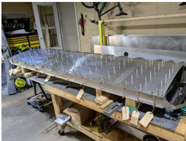
LH upper aft wing skin clecoed in place
