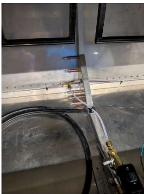
Brake system installation complete
