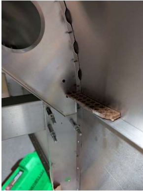
Wedge used to set vertical height of formers
