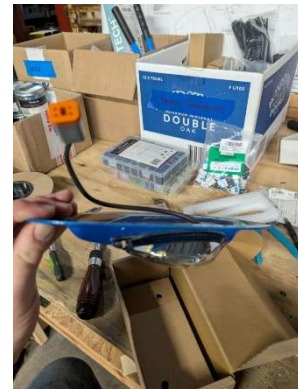
Installing DT connectors onto tip lights
