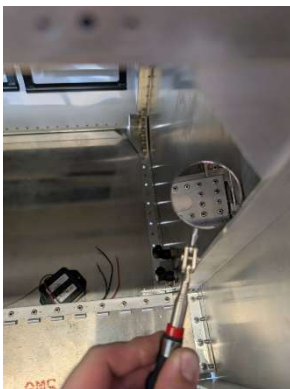
Panel cross tie rivets installed
