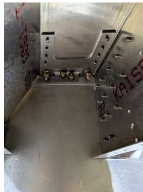
RH splice plate bolts
