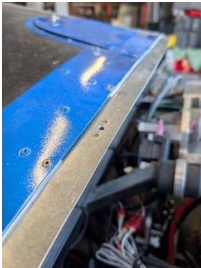
Nutplates installed in upper cowl shelf
