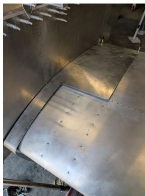
Marking offset trim line onto LH wing
