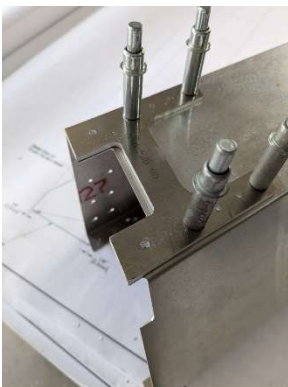
Cross tie splice located to drill pilot holes in crosstie box
