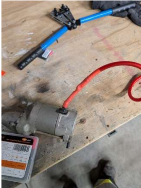
New starter cable crimped onto old cutoff
