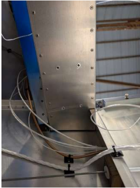
Rivnuts installed on bottom of cross tie box
