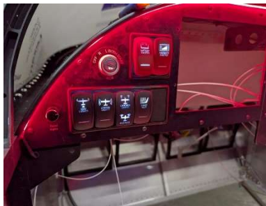
Main switch panel installed
