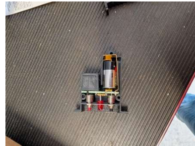
Battery and faceplate installed in RCPI
