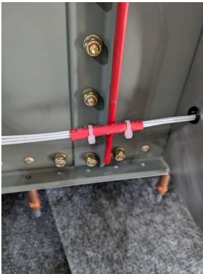
LH vertical stiffener area
