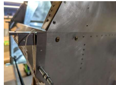
Bolts installed into upper splice plate
