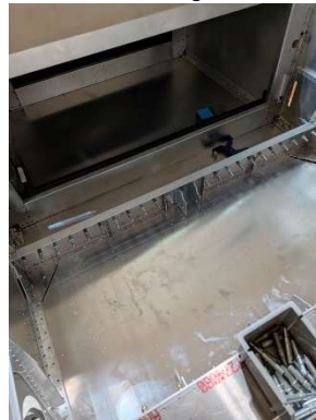
-02 assembly located and pilot drilled
