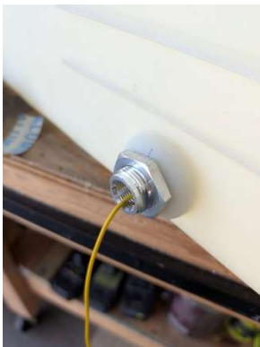
Main drain fitting fit
