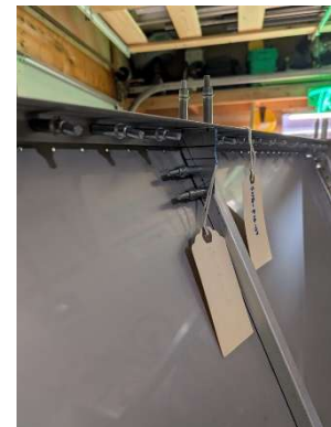
Firewall angle pilot drilled
