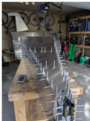
Aft fuselage floor located and pilot drilling in progress
