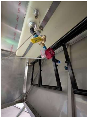
Installed another 45 and AN fitting in fuel run
