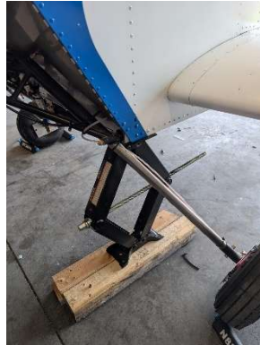
LH gear bolts replaced with NAS bolts
