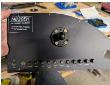
Circuit breakers installed
