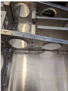
Final rivets installed in seat belt channels
