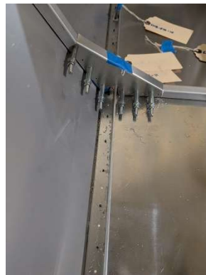
Gusset pilot drilled
