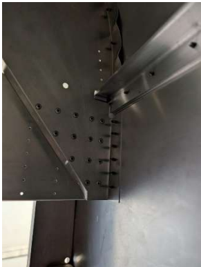
RH lower #1 former riveted to cross-tie box
