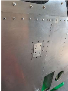
Vent assemblies complete
