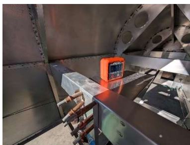
Mount secured to cross tie and leveled
